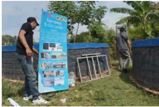
Gambar 7. Proses instalasi E-Ox Level
